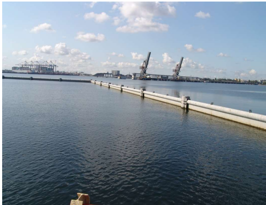
Permanent anti-spill barriers around the terminal
